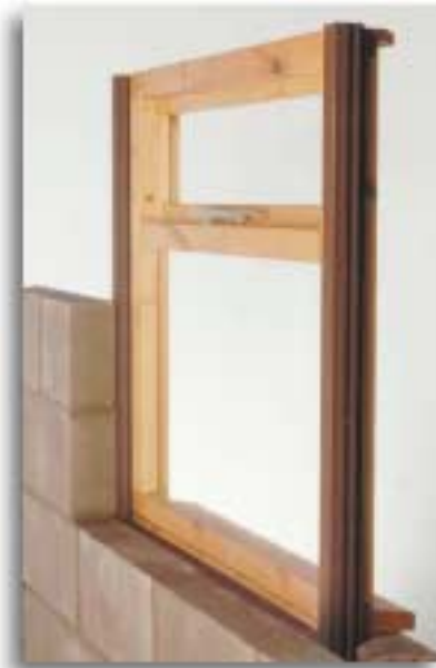
Wall built up around Thermabate
